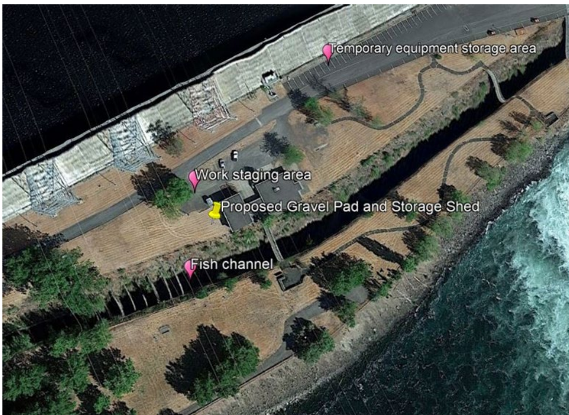
Figure 1. Close up of work area.
